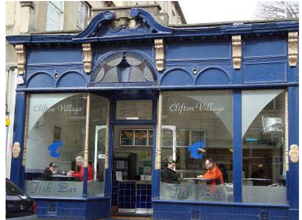
Figure 115: Elaborate timber shopfront, Princess Victoria Street
