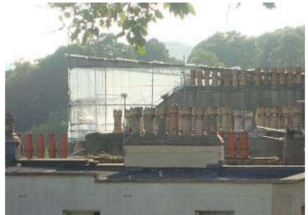
Figure 61: Chimney stacks and pots along the skyline
