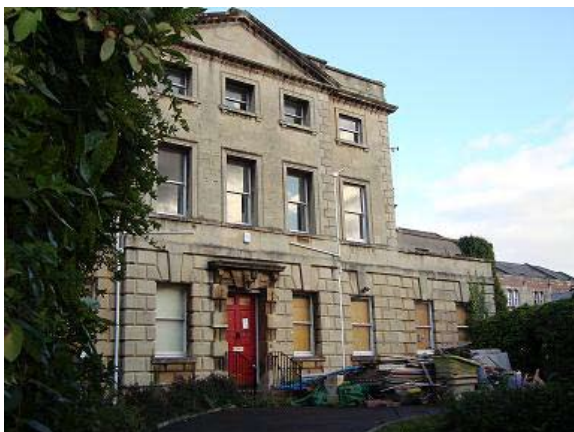
Figure 36: Mortimer House, Clifton Down Road
