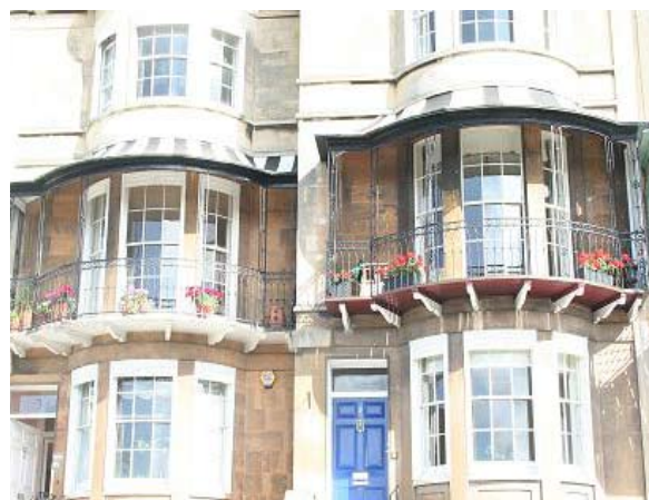
Figure 77: Bowed canopies, Sion Hill
