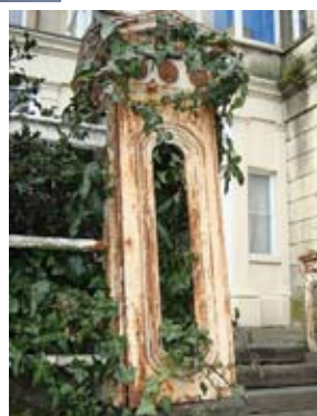
Figure 130-31: Examples of boundary rail- ings that have fallen into a severe state of disrepair and are at risk of being lost through irreparable damage
