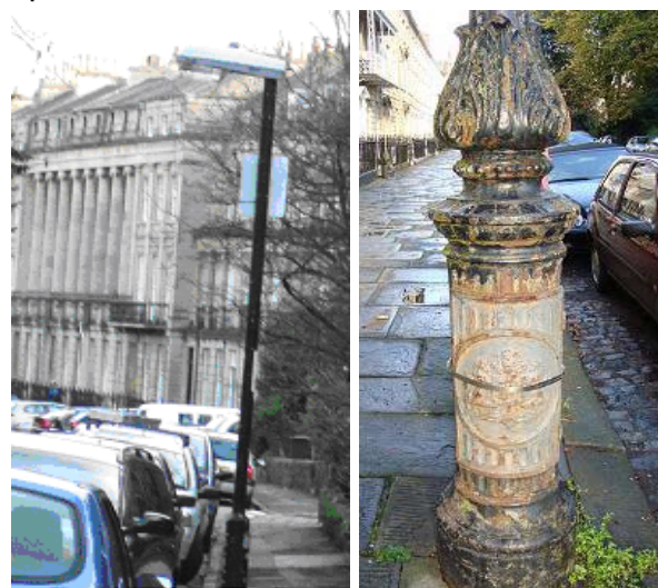
Figure 138-39: An unsympathetic modern replacement lamp standard adjacent to Grade II* Vyvyan Terrace and Christchurch; Grade II lamp standard in poor state of repair
