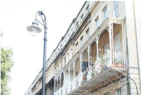
Figure 52: Balconies nos. 1-2 Caledonia Place
