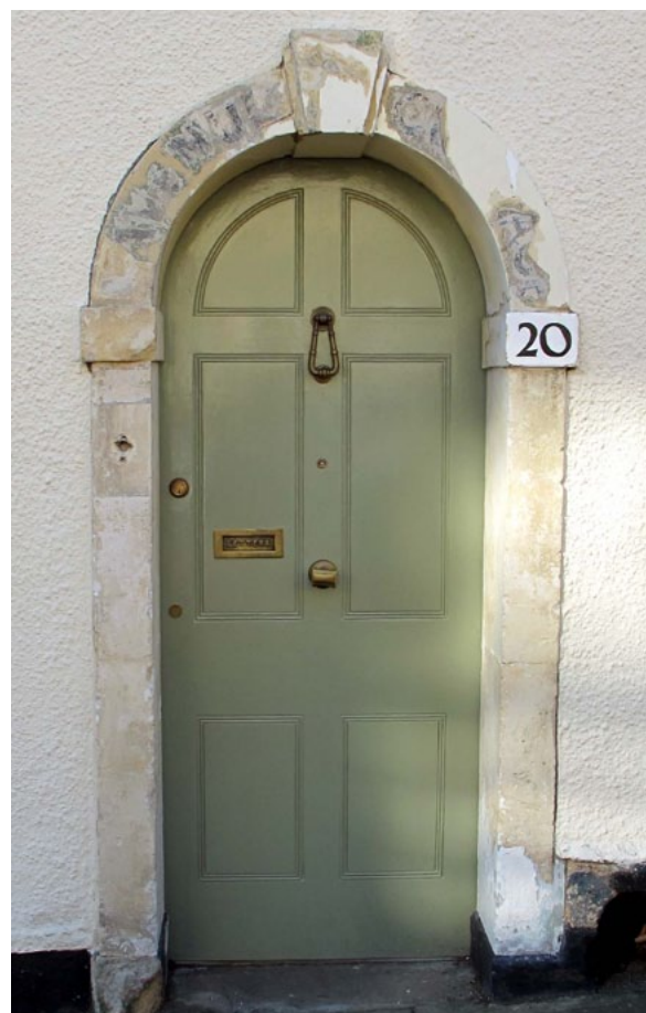
Figure 95: Flush-panel door with limestone surround, Luccombe Hill
