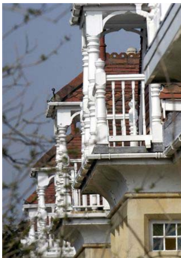
Figure 96: Timber balconies, Cotham Park
