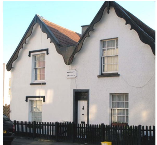
Figure 68: Woolcott Cottages, Lower Redland Road
