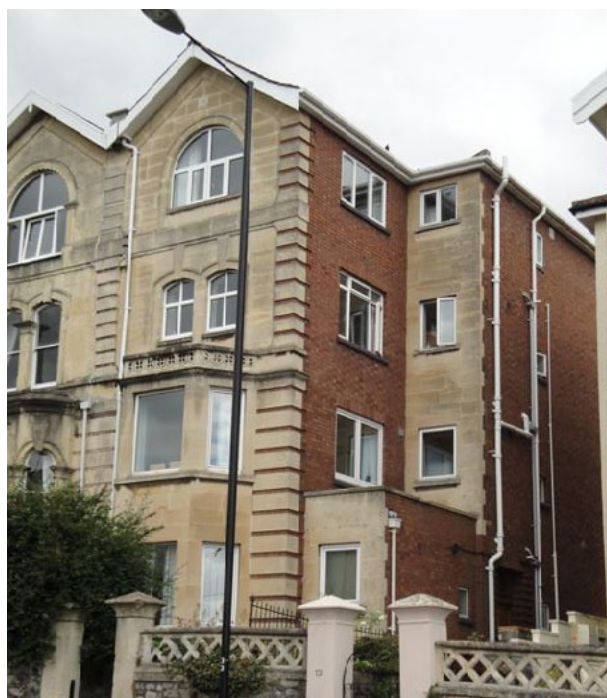
Figure 118: uPVC windows, Redland Road
