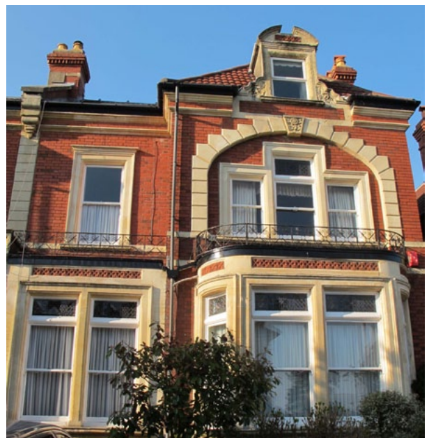
Figure 91: Late Victorian detailing, Woodstock Road
