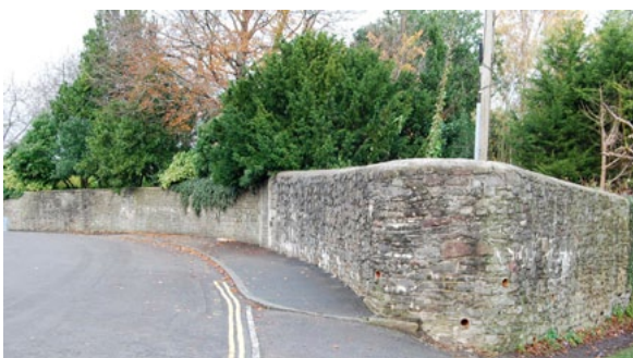
Figure 21: Boundary wall and private planting, Hartfield Avenue
