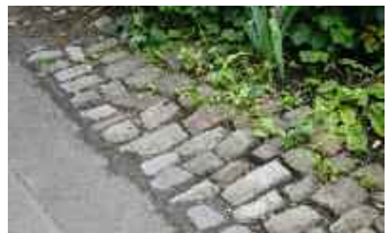
Figure 66: Traditional setts overlain with tarmac
