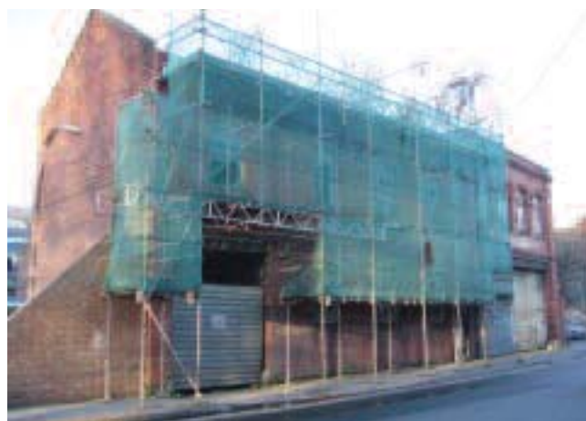
Figure 39: Early 20th century warehouse on Unity Street, with no roof the fabric of the building is deteriorating rapidly
