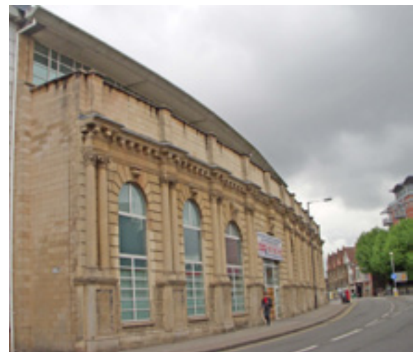
Figure 28: Retained facade of former Coliseum
