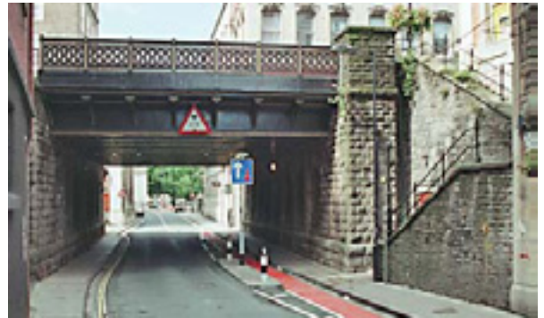
Figure 22: Park Street Viaduct viewed from Frogmore Street
