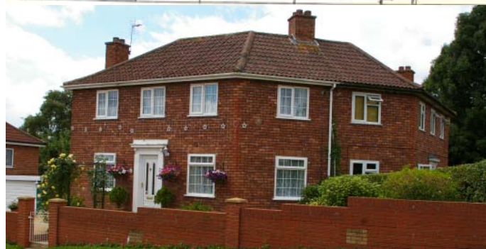
Figure 66: CBA5 type (Original drawing ©BRO) uPVC windows, g-f windows of left house have top hung vents, f-f side-hung casements & glazing bars give some character. Shutters lost
