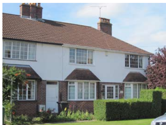
Figure 77: St Edyth's Road type (Original drawing ©BRO photo ©John Roberts) uPVC windows, although the means of opening and glazing bars maintain some of the character
