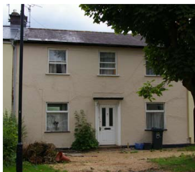
Figure 64: DLC5 Timber first floor sash windows, ground floor windows uPVC with out of character top hung vents and no glazing bars, timber door. Shutters lost
