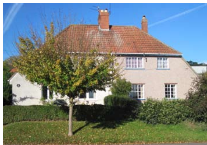
Figure 70: HBA5 type (©John Roberts) House on right is a very good example with original metal windows. House on left has uPVC windows with no glazing bars. End chimney stack lost
