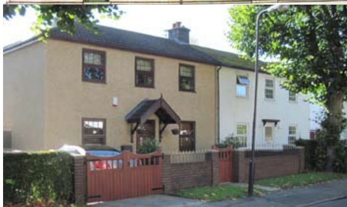
Figure 60: DLA5 type (Original drawing ©BRO photo ©John Roberts) Windows now uPVC top hung casements with wide meeting rails, although the glazing bars maintain some character. Replacement doors. Shutters and end chimney stacks lost. House on left has out of character pitched canopy over door
