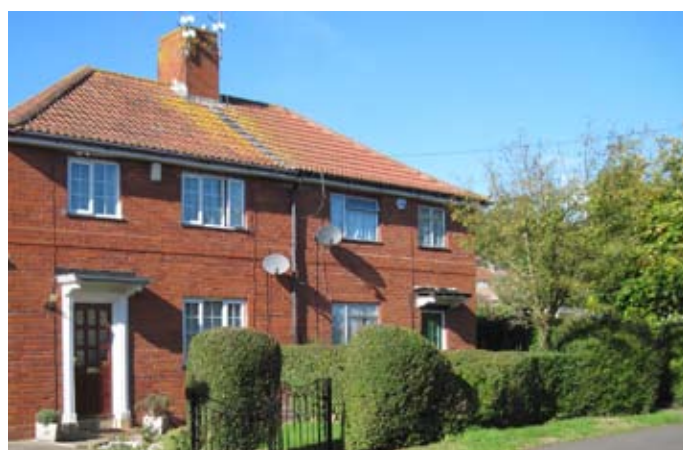
Figure 72: MGD2 type (Original drawing ©BRO photo ©John Roberts) Both houses have uPVC windows. The side hung casements and glazing bars of left-hand house maintain some character, but house on right has out of character casements with no glazing bars
