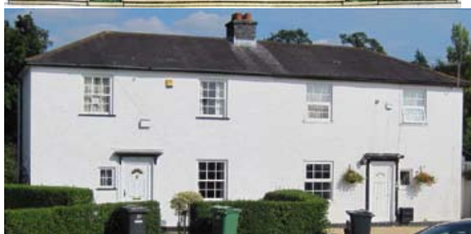
Figure 59: DLA2 type (Original drawing ©BRO photo ©John Roberts) House on left is a good example with original timber sash windows; house on right has uPVC top-hung casements with wide meeting rail, although the glazing bars maintain some character. Out of character doors. Shutters and end chimney stacks lost
