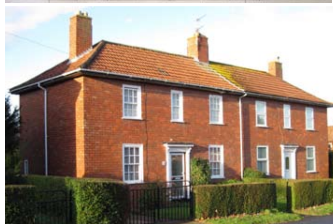
Figure 69: CNA5 type (Original drawing ©BRO photo ©John Roberts) House on left is a very good example with original timber sash windows. House on right has uPVC windows with no glazing bars. Both doors are out of character. Shutters lost
