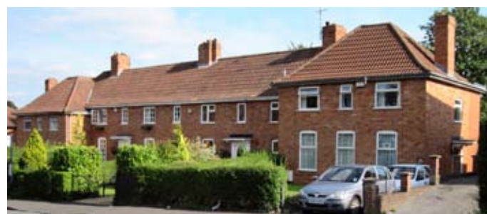
Figure 73: WDA5 type (Original drawing ©BRO photo ©John Roberts) Shows WDA5 “stepping down” the hill of Westbury Lane. The house to the immediate left of centre is a very good example with both original timber windows and door. All other windows are uPVC with out of character means of opening and without glazing bars
