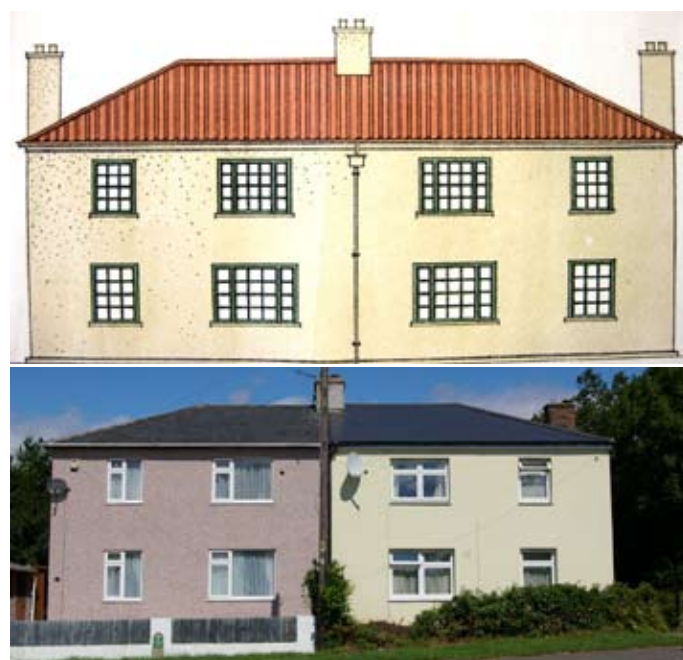
Figure 61: DLA6 type (Original drawing ©BRO) All windows uPVC casement windows with no glazing bars. End chimney stacks lost. House on left has pebble-dash pinkish render
