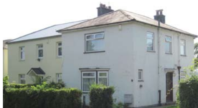
Figure 65: DLD5 type (Original drawings ©BRO photo ©John Roberts) All windows uPVC with top hung vents and no glazing bars. House on left has been overclad with loss of original door surround, replaced by a pitched canopy
