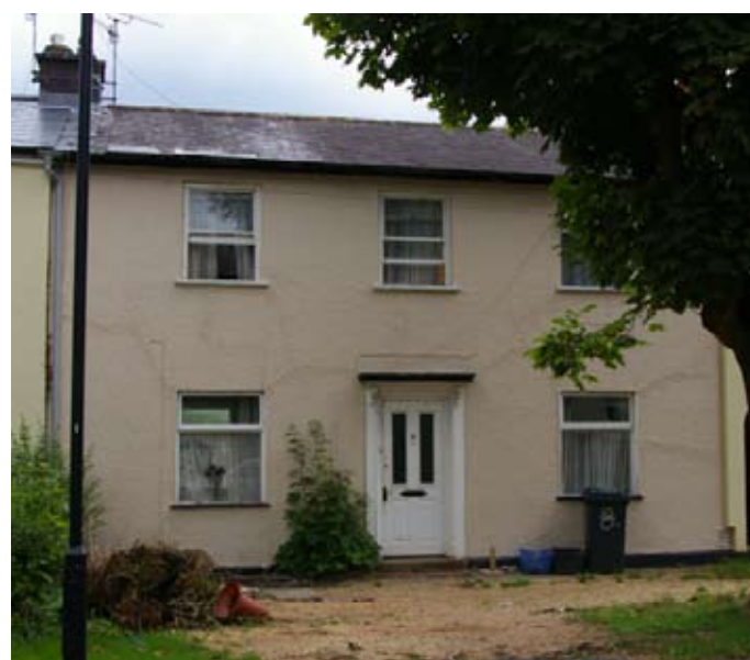
Figure 64: DLC5 Timber first floor sash windows, ground floor windows uPVC with out of character top hung vents and no glazing bars, timber door. Shutters lost
