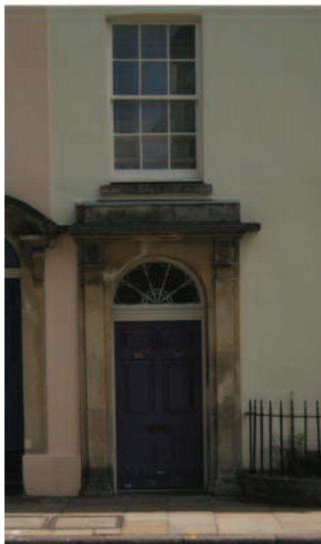
Figure 34: No. 96 St Michael's Hill: Typical Georgian window and door details: six-over-six timber sash window; six panel door with decorative fanlight and Lime stone door surround
