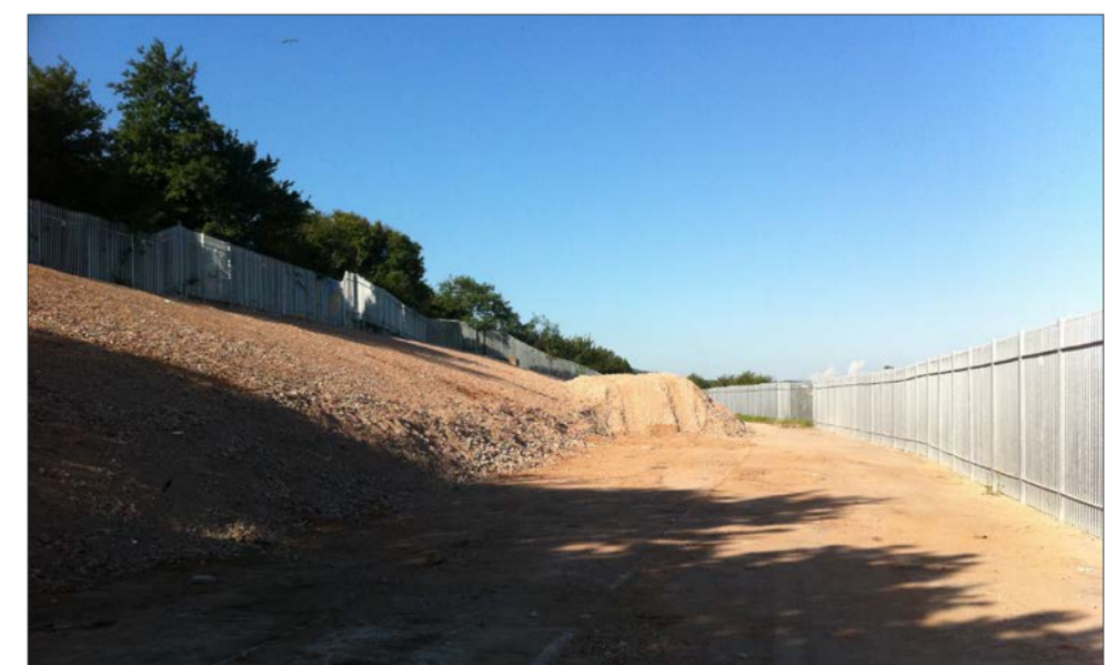
Photo of made up ground
