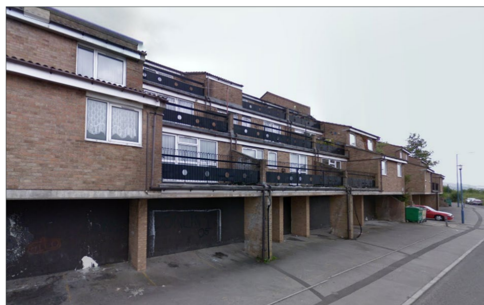
Photo of demolished building on site
