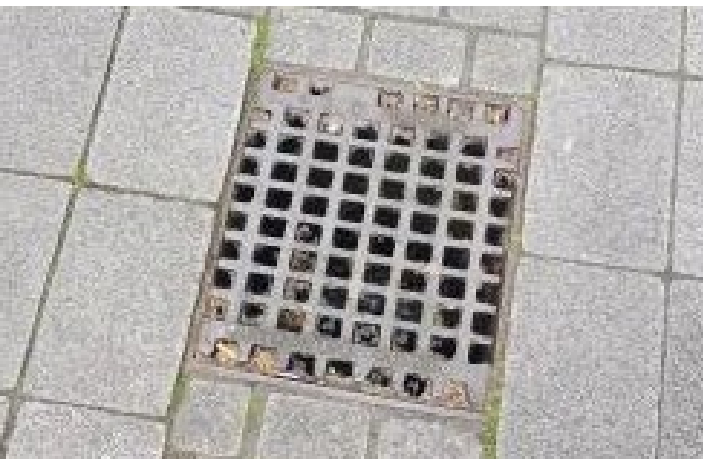
Fig 3: Heel guard gully cover in footway
