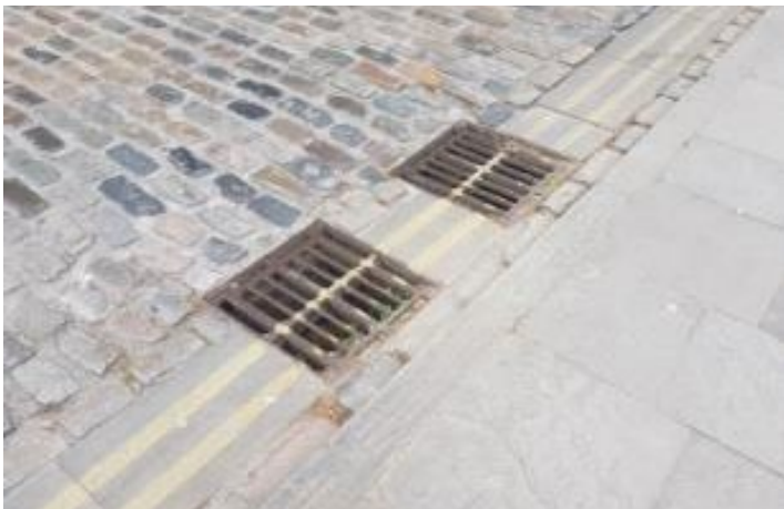
Fig 3: Heel guard gully cover in footway
