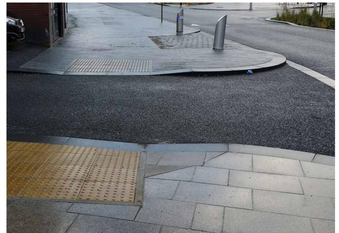
New safer crossing with tactile paving and narrower road carriageway to cross
