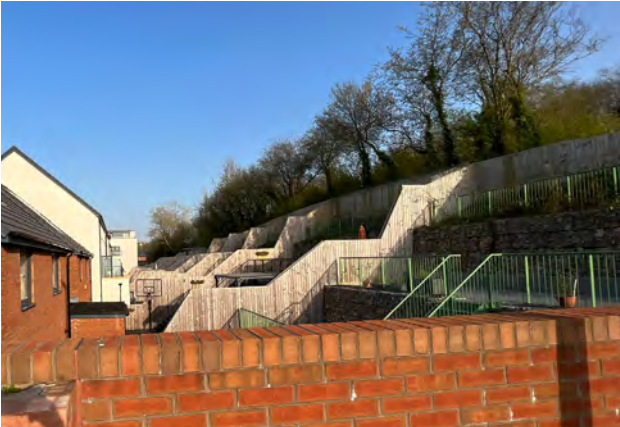
Sidford Road - Terraced gardens with gabion walls.
