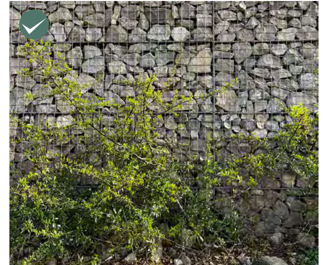
High-quality gabion retaining wall with additional planting
