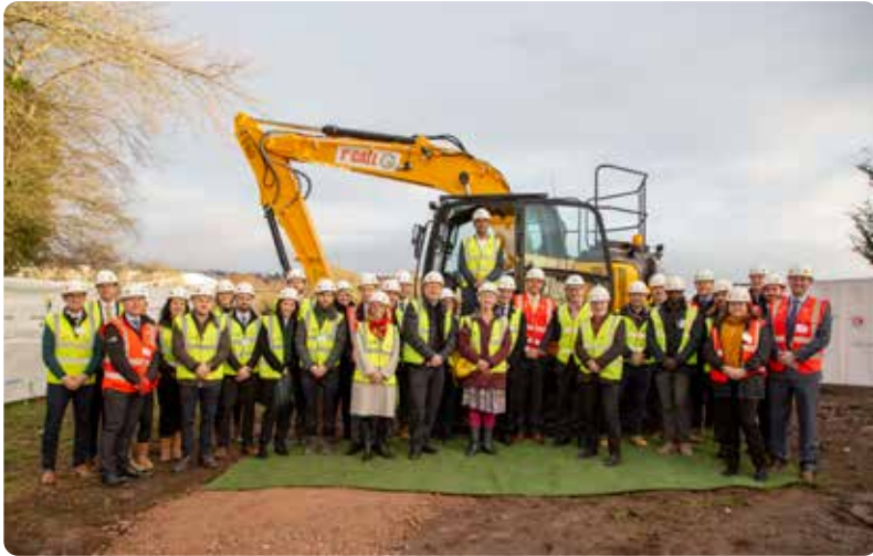
Ground-breaking event at Ashton Rise with the Mayor, Housing Delivery Development Team Manager and Willmott Dixon Construction Ltd.
