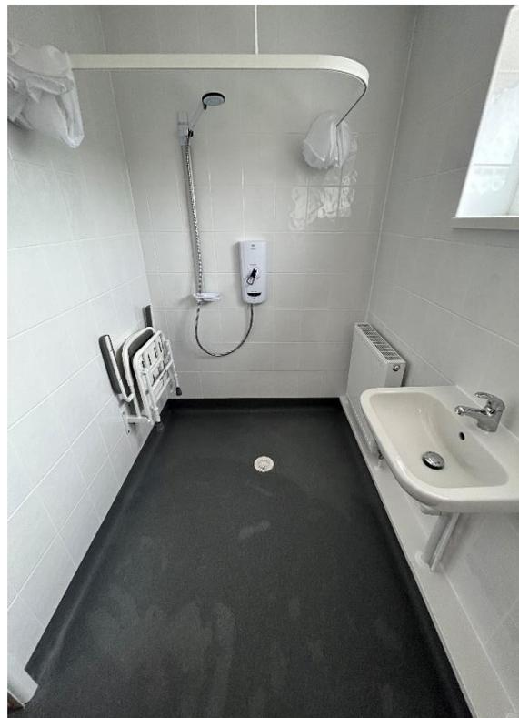
**Electric Showers** will be high quality thermostatic controlled showers with an adjustable riser and a 2m long shower hose where assisted showering is required.
