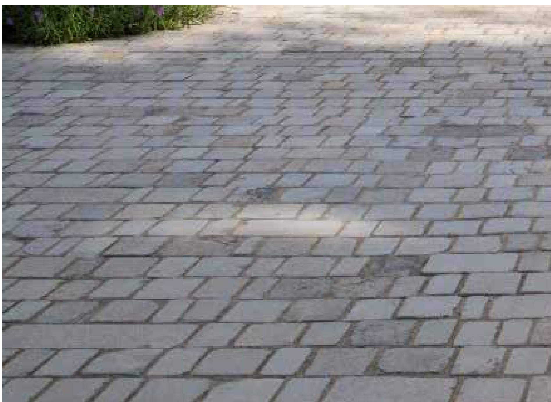
New high quality pennant stone block paving will replace the existing tarmac at the entrance to St George's Park
