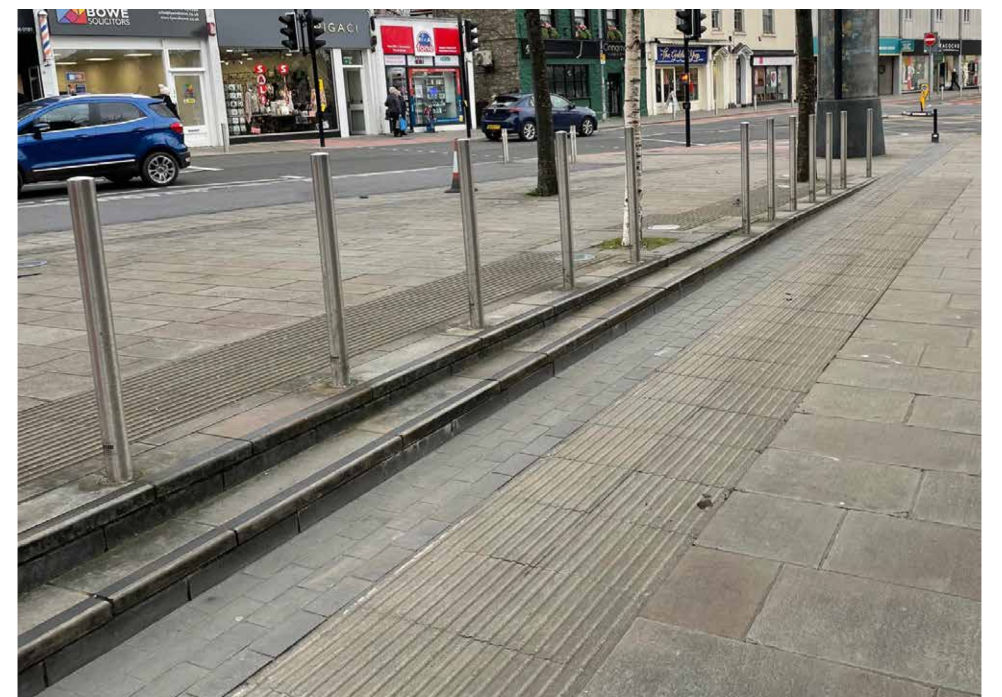
Steps that taper and gentle slopes will be created to deal with the change in level between the shops to the east and the square itself. The steps will have tactile paving on both sides.
