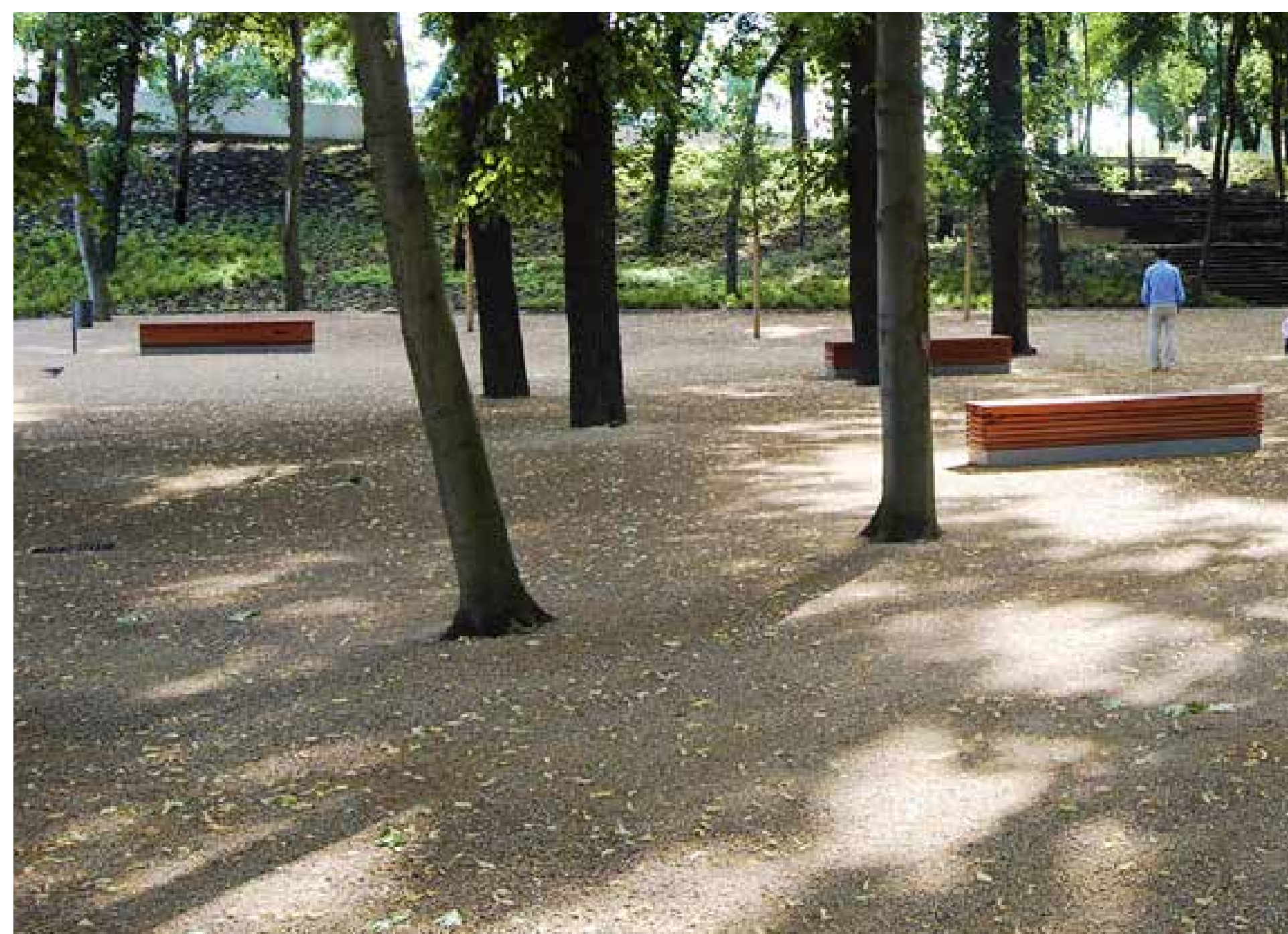
Use of flexible paving around the trees in the middle of Stockwood Square will cover raised tree roots & create a safe, even surface
