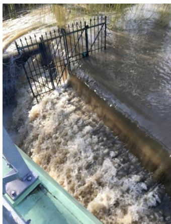
Plate 1. Overtopping at Bathurst Basin.
