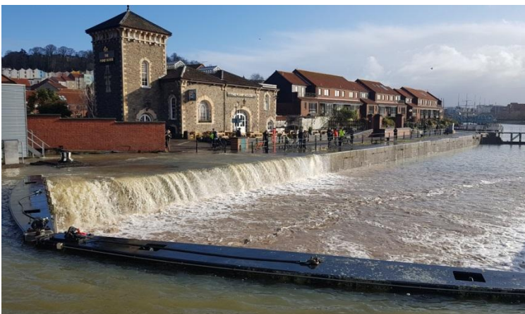
Plate 2. Overtopping at Junction Lock (Cumberland Basin).
