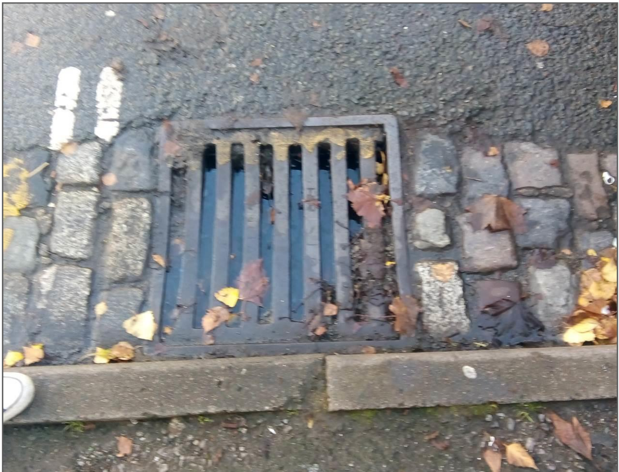
Plate 4: A blocked gully within the flood investigation area on Cheltenham Road, taken on the 30 th November 2018.
