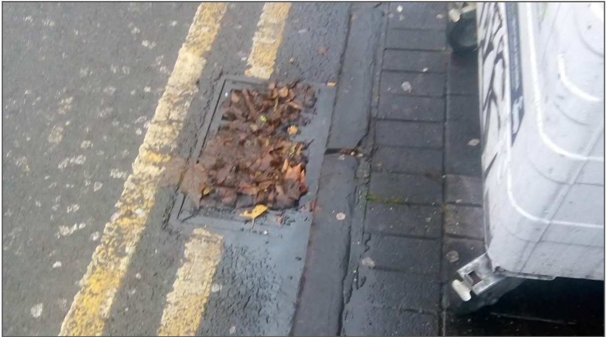
Plate 3: A blocked or blinded gully within the flood investigation area on Cheltenham Road, taken on the 30 th November 2018.
