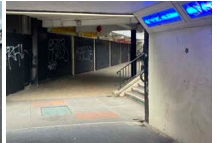
Subway ends in area with limited inter-visibility
