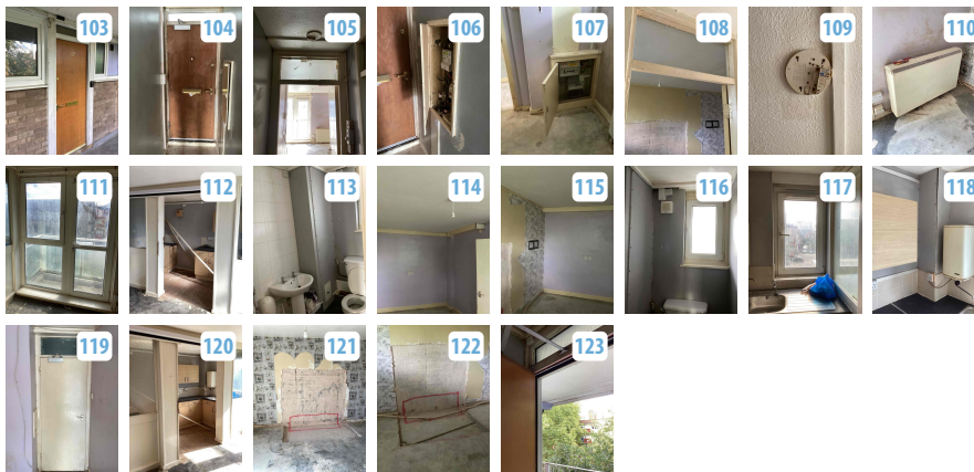
LOCATION Void flat 17, 17/9/2024
